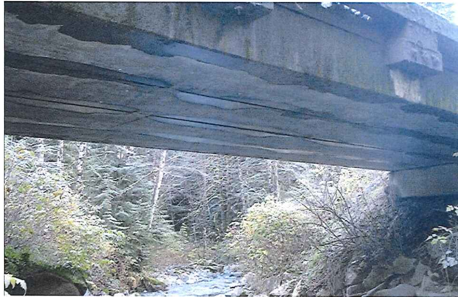
CK2094 Crossing upstream
