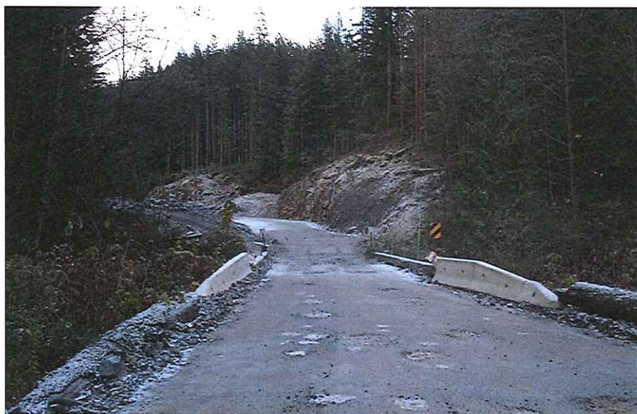
CK2094 Approach Right Bank
