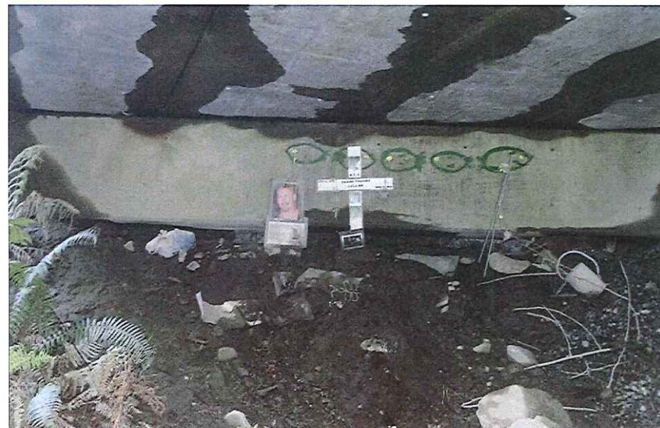
CK2094 Abutment Left Bank
