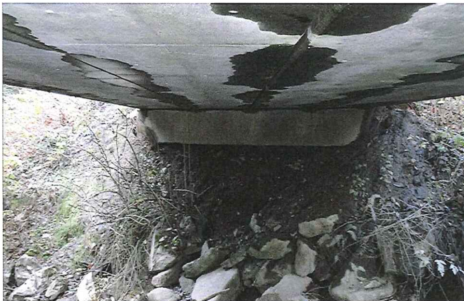
CK2094 Abutment Right Bank
